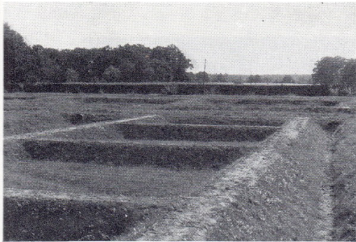
Fig. 197 Dubisch spawning ponds before filling with water. Fence made of reeds placed round the ponds for protection against wind and cold. Milicz, Wroclaw, Poland.
